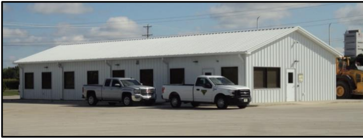
Above is a picture of the Smith Ready Mix administration building. It houses the man/computer control station, the dispatcher and other company offices
